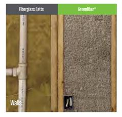
Greenfiber cellulose insulation fills cavities from side-to-side and top-to-bottom, without gaps or voids around obstructions like blocking or bridging, and it fits tightly around wiring or electrical boxes within the cavity for a Grade-1 install that blocks sound and resists air infiltration.
